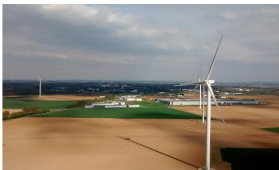
Wind turbines at the wind farm in Roye, department of Somme, Picardie region
